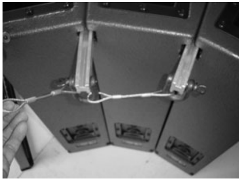
(3) Safety steel detail (top)
